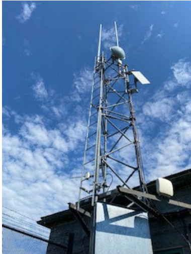
Figure 1. Existing Nash Hill Tower
