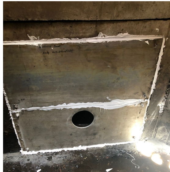
Figure 2: One of Two Six-Inch Restricted Stormwater Connections
